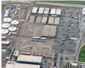
Bran Sands enhanced AD Plant – 35,200tds/y, 4MWe enhanced AD plant
