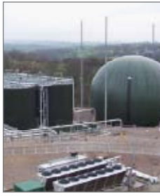
Blackburn Anaerobic Digestion Plant – 740m 3 /d, 2MWe Blackburn enhanced AD plant - 740m 3 /d, 2MWe
